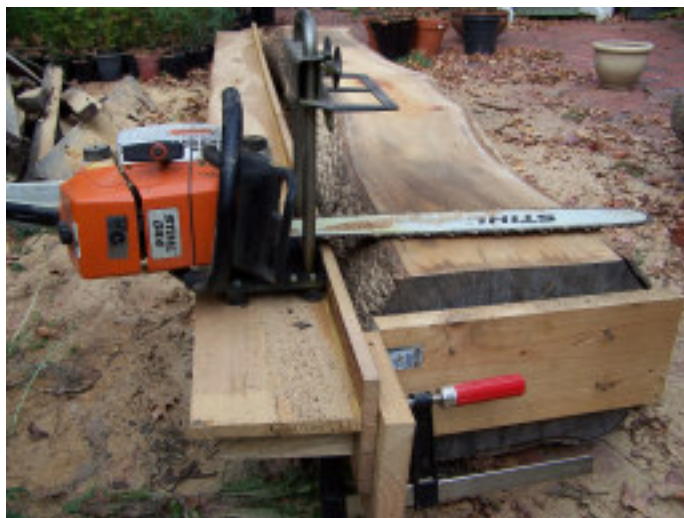
The first cut: the timber guide is fixed in place using two end brackets
